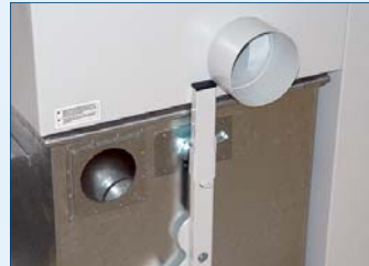
Intake pipe DN 140 and inspection glass in collection tank
